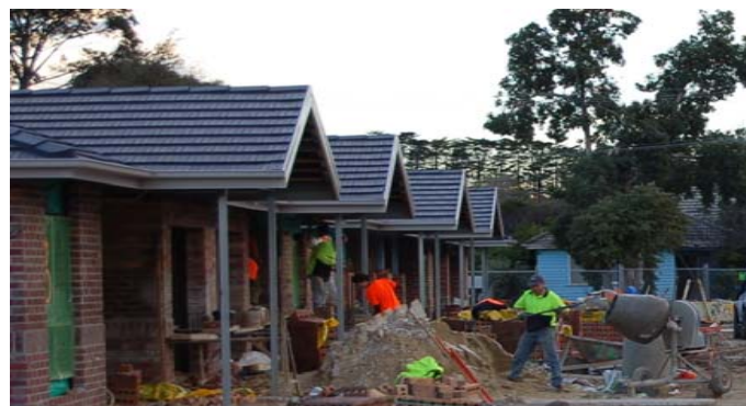
Above: Villa Units at Corpus Christi Village under construction.
